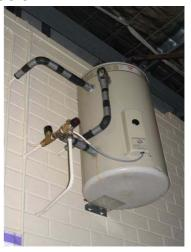
Figure 7 Pipe insulation on electric HWS
